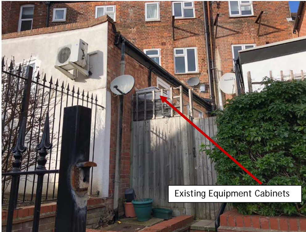
View of rear of building
